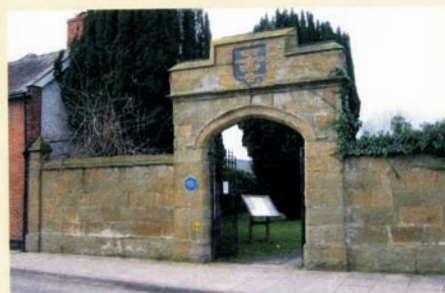
The stone entrance to St Leonard's churchyard, off Corve Street north of the town centre, constructed in the 19th Century utilising stone from the demolition of a Carmelite Monastery which once occupied the site.
