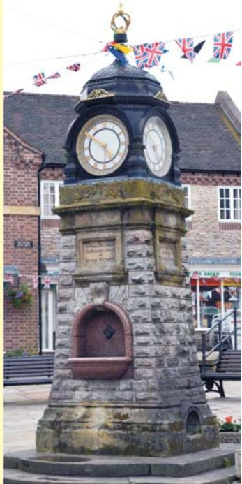
This shows three different stone types. The bulk of the structure is in local Wenlock Limestone, cut into regular blocks but with a rusticated finish. Many blocks contain fossil corals as well as crinoids (*below*).
