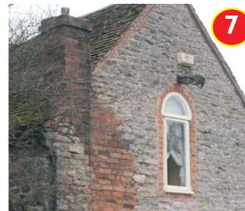
There are many examples of brick-built flues and chimneys, because heat breaks down limestone.
