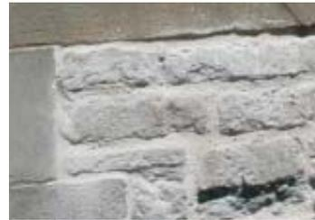
Wenlock limestone, with its more clearly layered structure, can be cut only into smaller rough blocks.
