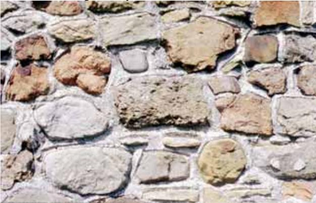
**Figure 6.** Geological mixture in Norman wall, Cardington Church.
