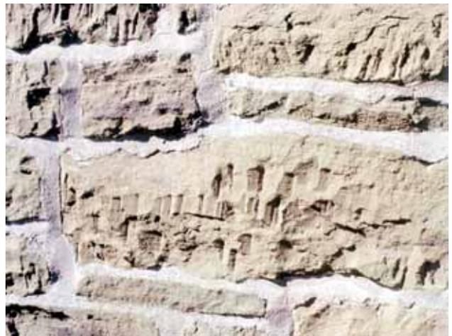
**Figure 9.** Rushbury Church, revealing Soudley Sandstone with 19<sup>th</sup> Century tool marks - 'rustication'.
